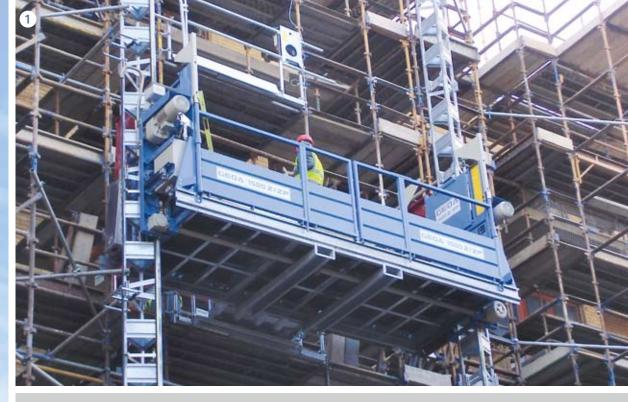
Your powerful partner for heavy loads and efficient work methods. Numerous different platform versions mean the unit can be employed to optimum capacity on all construction sites.
