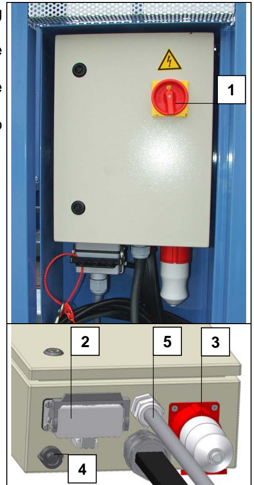
Fig. 14 Cable box switch cabinet
