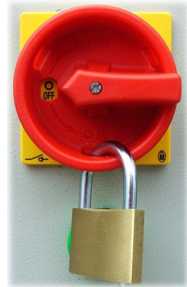
Fig. 62: Main switch secured
