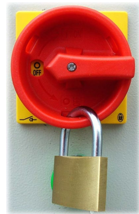
Fig. 44: Main switch secured
