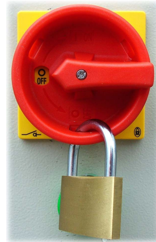
Fig. 29: Securing the main switch
