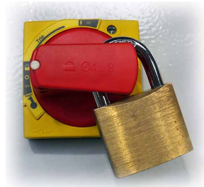
Fig. 44 Securing the main switch
