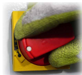
Fig. 61 Resetting the circuit breaker
