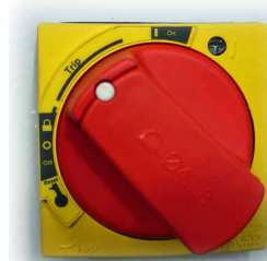
Fig. 60 Circuit breaker tripped
