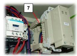
➤ Insert the car control into the plug-in device (7).
